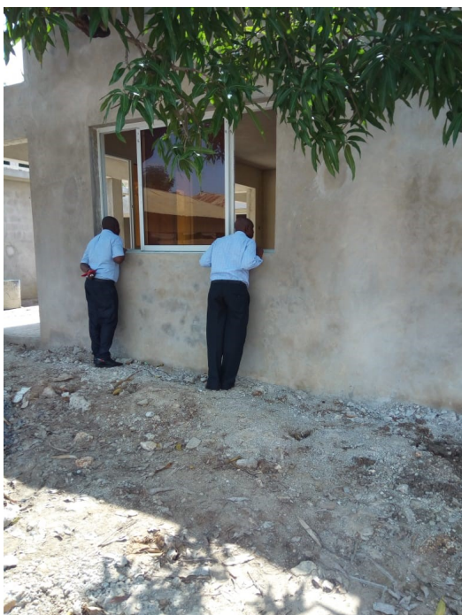
Inspecting the new classrooms. June 2018
